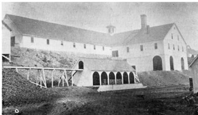
The first smelter in the Pacific Northwest was built at Ketchum in the fall of 1881. This picture of smelter and bullion shed was taken in 1883.
